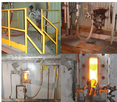
Figure 7. Typical stationary liquor gun assembly
