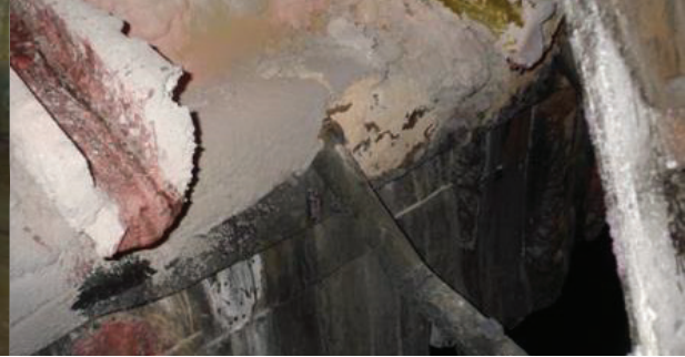
Figure 2. Large opening below spouts and dried smelt covering internals and smelt spout
