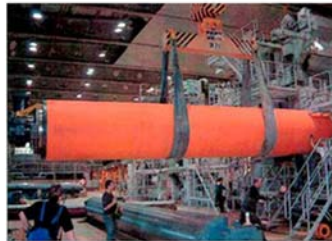
Suction roll installation
